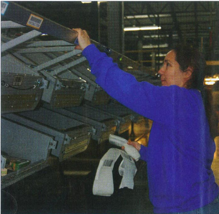
Lights at the end of the chute tell operators proper carton size, along with order information.
